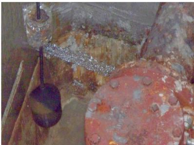
*Figure 1. Vault Water Infiltration*
